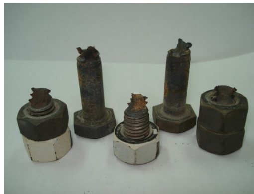
Figure 22. Bolt and nut failure
