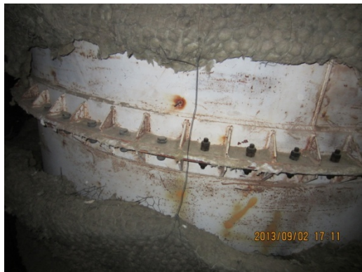
Figure 29.one by one methods bolt renew
