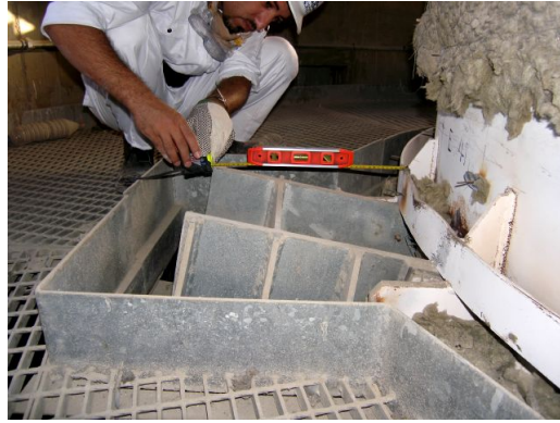
Figure 9. Stack fall down
