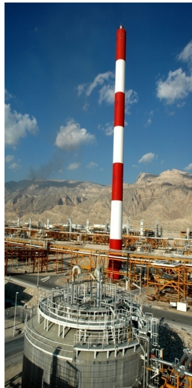
Figure 2.sulfur recovery units stack
